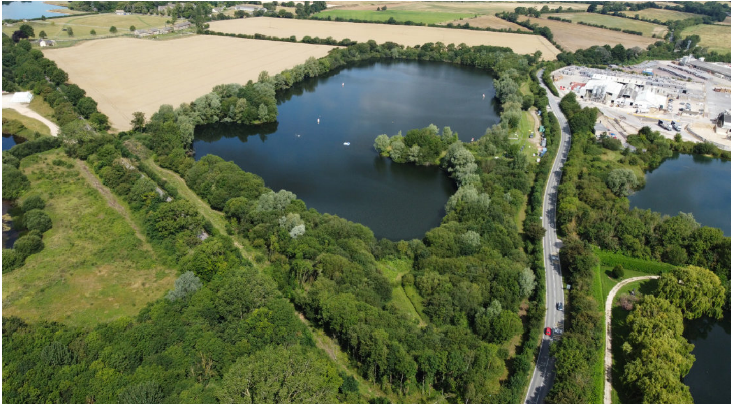
Aerial view of the site from the South East
